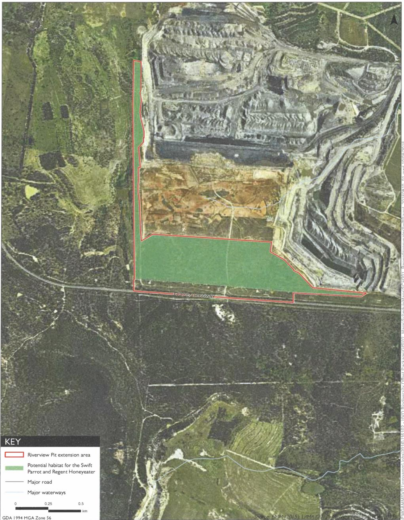
Potential Regent Honeyeater and Swift Parrot habitat in the Riverview Pit extension area Hunter Valley Operations - State-approved mining Schedule 2
